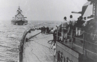
Crewmen aboard PRINZ EUGEN pass a light line to BISMARCK prior to sending either a fuel line or a tow line to the battleship. This maneuver was practiced in the Baltic prior to RHEINÜBUNG. Passing lines at sea was performed in case either ship became disabled or lost fuel during their planned sortie. Admiral Günther Lütjens commanded RHEINÜBUNG from aboard BISMARCK. (NHC)
