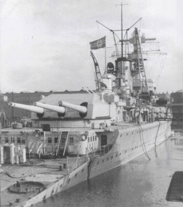
The Germans took measures to reduce LÜTZOW's aft weight when she arrived back at Kiel on 12 April 1940. This sufficiently restored trim for her to enter drydock at Deutsche Werke. Lightening measures included removing both quadruple torpedo mounts on her fantail. The base ring for the starboard torpedo mount remains on the deck. The hull break that resulted from the British torpedo hit occurred right at the armor belt's aft end. (Bundesarchiv)
